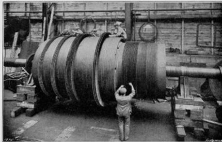
Fig. 21. Blading a Rotor at the Turbina Works.
