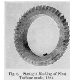
Fig. 6. Straight Blading of First Turbine made, 1884.
