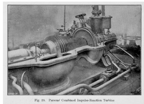
Fig. 29. Parsons' Combined Impulse-Reaction Turbine
